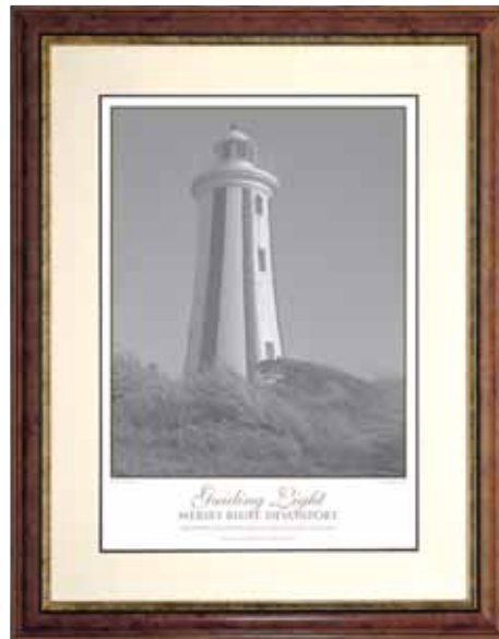
Guiding Light Mersey Bluff, Devonport Constructed at Devonport Tasmania in 1889 at a height of 13 metres.
